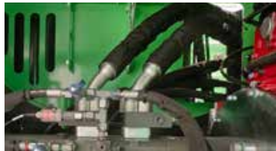
All high pressure hydraulic hoses in the engine compartment are secured in sleeves to protect service personnel.
